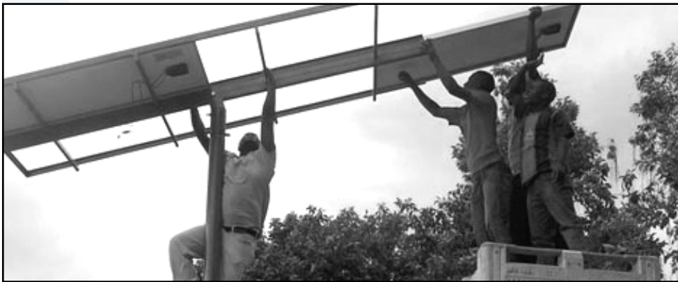
Workers install solar panels at water treatment facility.
